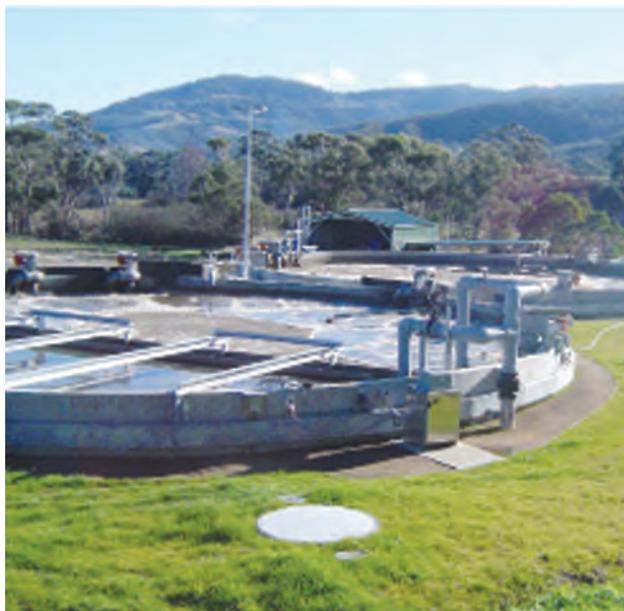
The PWTech Hybrid Biological Nutrient Removal (HBNR) process typically employs a twin circular tank design. The first tank (foreground) is an aerobic-anoxic tank (AAT). The second tank (background) is an intermittently operated clarifier (IOC).
